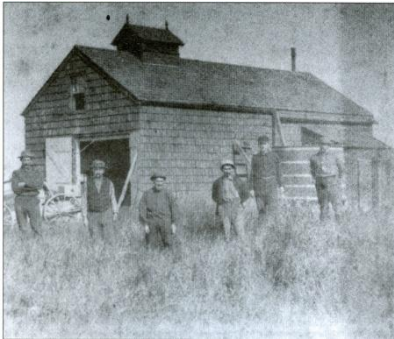
This 1871 style station or "Red House" named because of its exterior color 42ft long x 18 ft wide with 4 rooms
